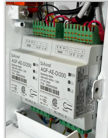
Factory Installed aGate Meter 1 and Meter 2
